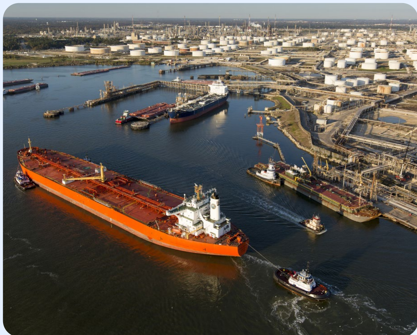
Above: Houston Ship Channel. Photo courtesy of ExxonMobil/Robert Seale
